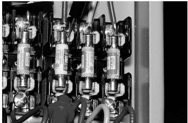
Figure 11. Fuse Test - Volt Meter Method
