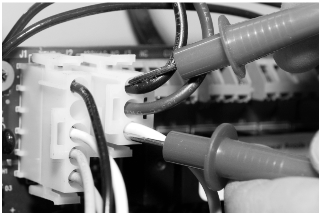
Figure 47. Checking for 120 VAC Power
